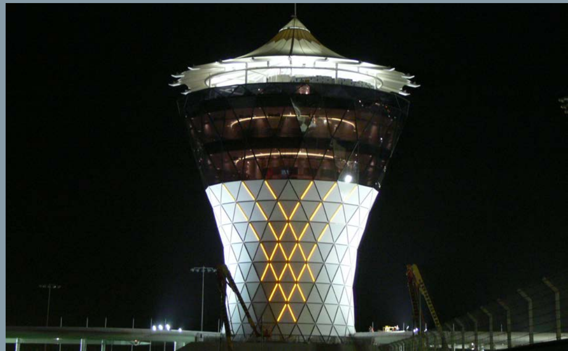
Sun Tower, Yas Marina Formula One Racing Circuit: Replacing aluminum panels
