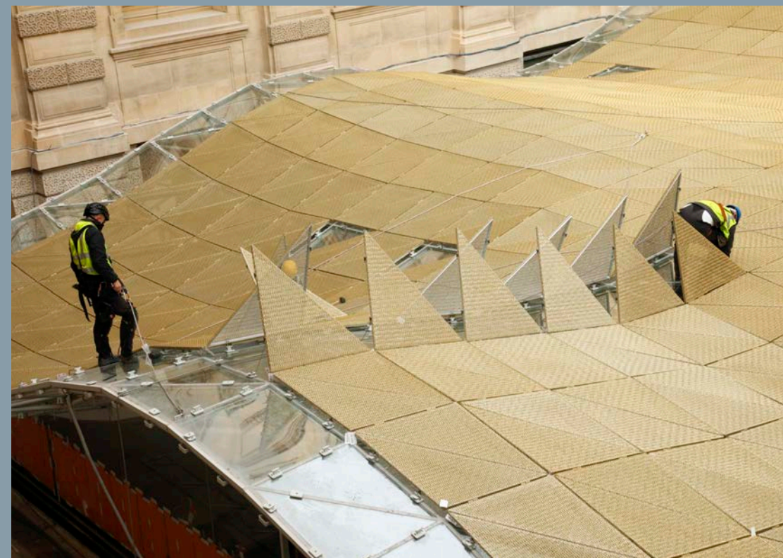
Musée du Louvre, Paris: Inspection and maintenance. Photo by Trevor Palin
