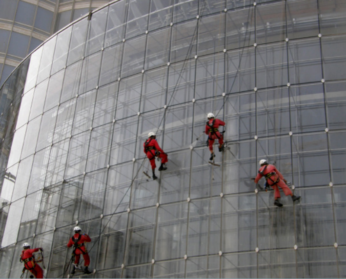
Burj Khalifa: Façade climbers inspecting silicon joints
