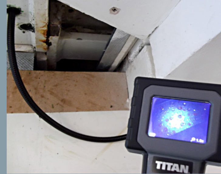
Locating the source of a water leak with an endoscope camera
