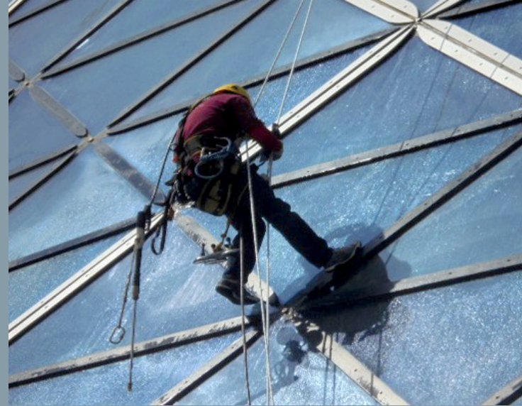
Adnec Tower/Capital Gate: Water leakage test
