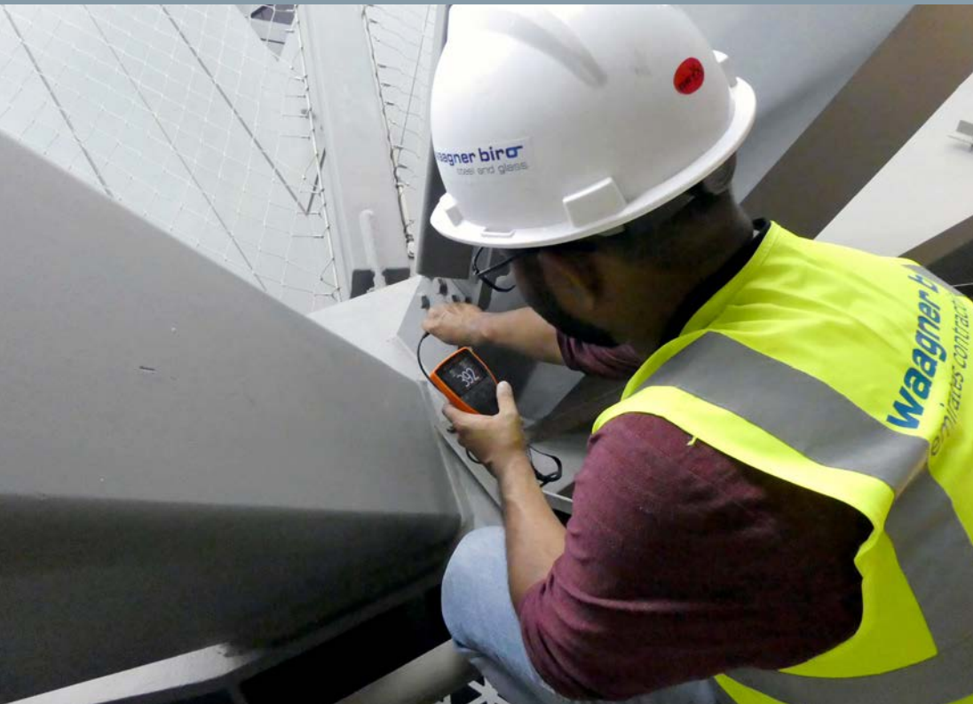
Louvre Abu Dhabi: Inspecting the paint for corrosion for preventative maintenance-recommendations
