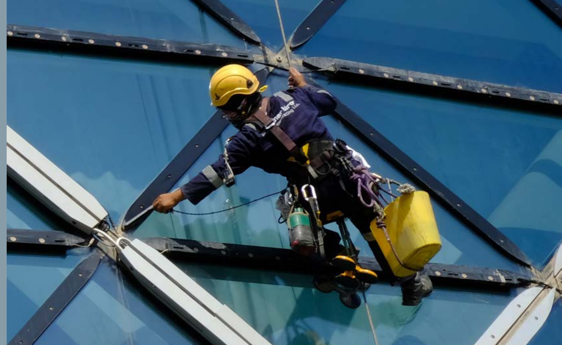
Adnec Tower/Capital Gate: Inspection and preventative maintenance
