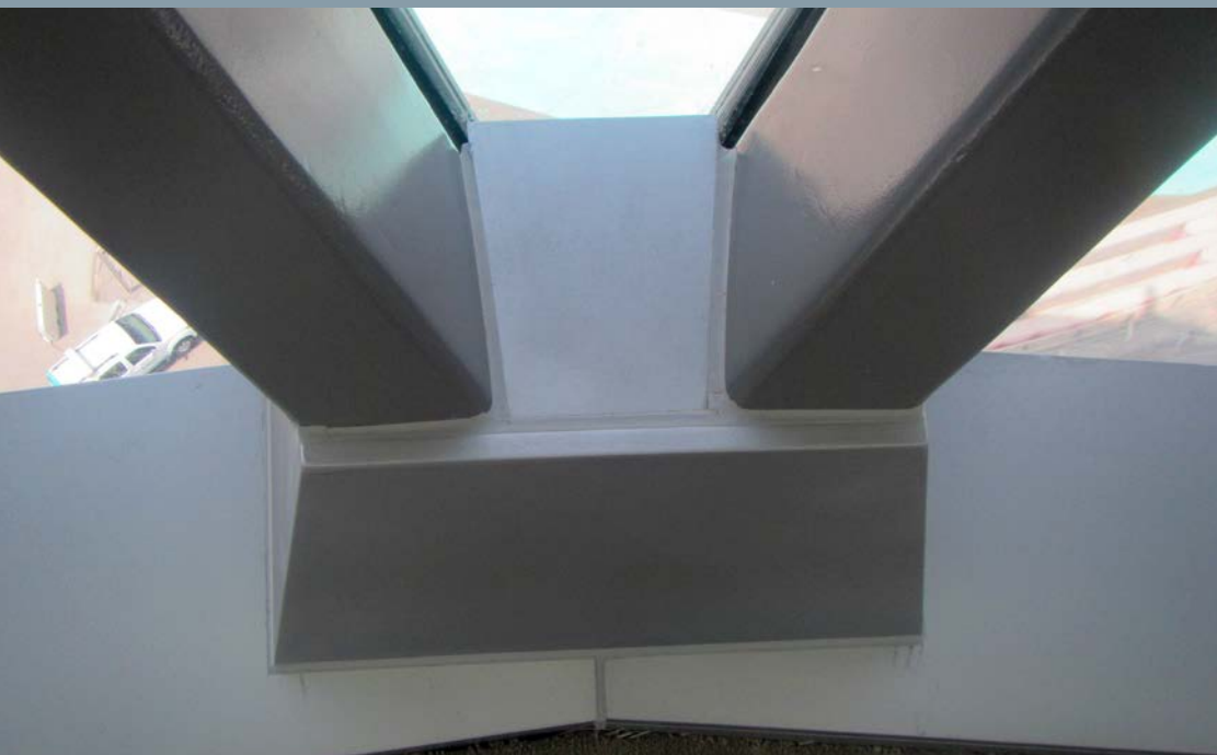
Yas Racetrack Shams Tower: Final application of corrosion protection of existing structure
