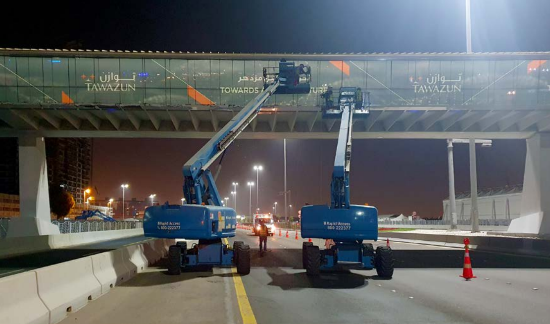
Yas Marina Bridge: Traffic management
