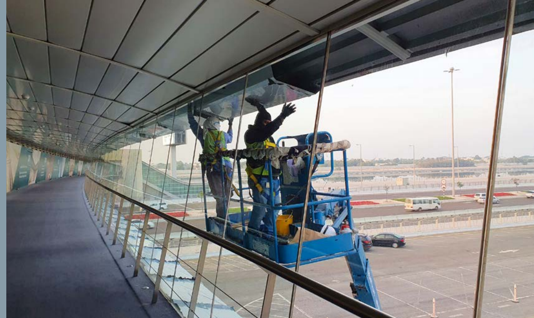
Yas Marina Bridge: Replacing aluminum panels
