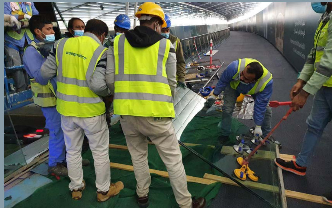
Yas Marina Bridge: Replacing glass panes
