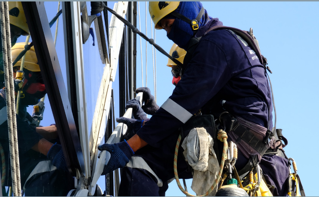
Adnec Tower/Capital Gate: water tightness inspection
