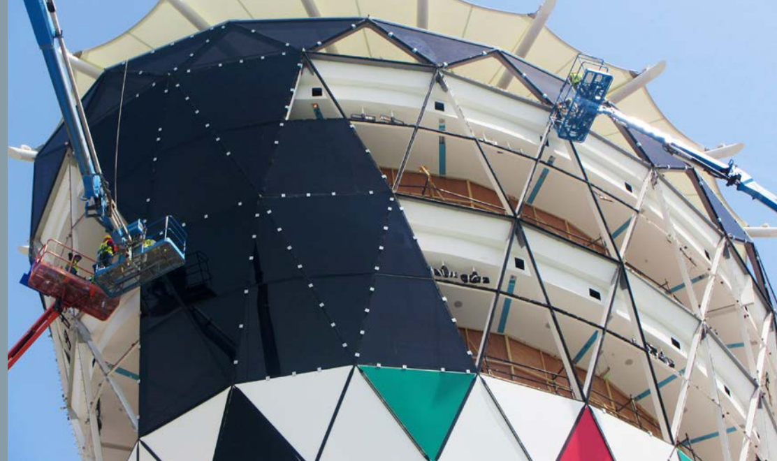
Sun Tower, Yas Marina Formula One Racing Circuit: Glass replacement, LED-installation
